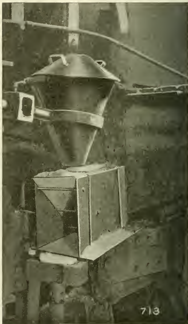
FIG. 3. CRUCIBLE AND MOLD BOX IN POSITION FOR WELDING MUD RING.
